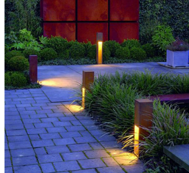
Low level Bollard Lighting to Paths
